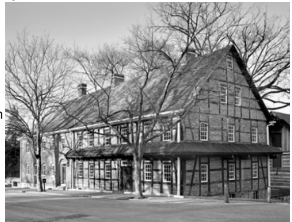
Single Brothers House at Old Salem, restored in 1964 to its 1769 condition (brick addition, 1786). Photograph by Tim Buchman. Courtesy of Preservation North Carolina.
